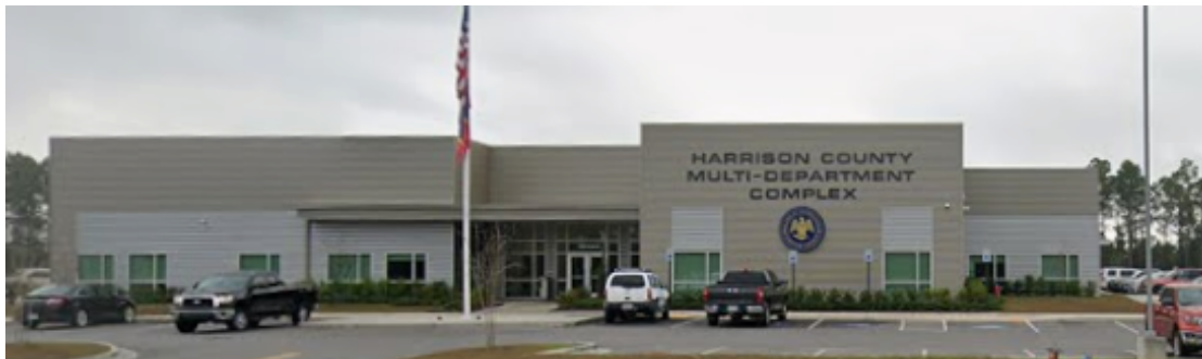
Harrison County Multi-Department Complex, 1 Seaway Rd, Gulfport, MS 39503
